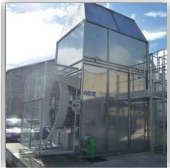
All the mechanical components to be maintained are located at man height, out of the wet air flow.
